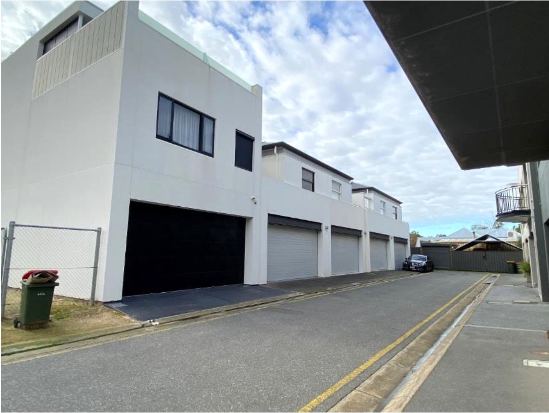
Photo 3.3 – development on northern side of Watson Street
