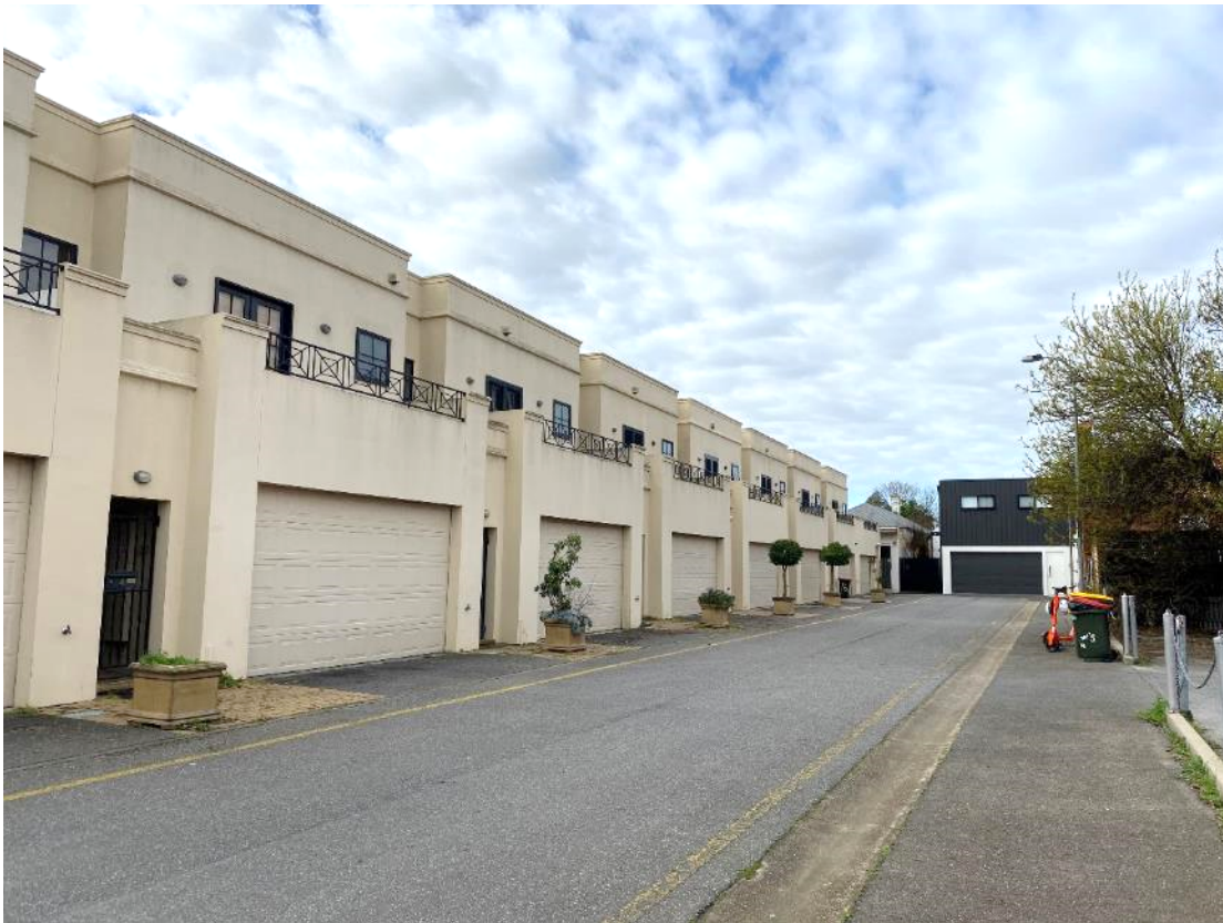
Photo 3.4 – development on northern side of Stephens Street
